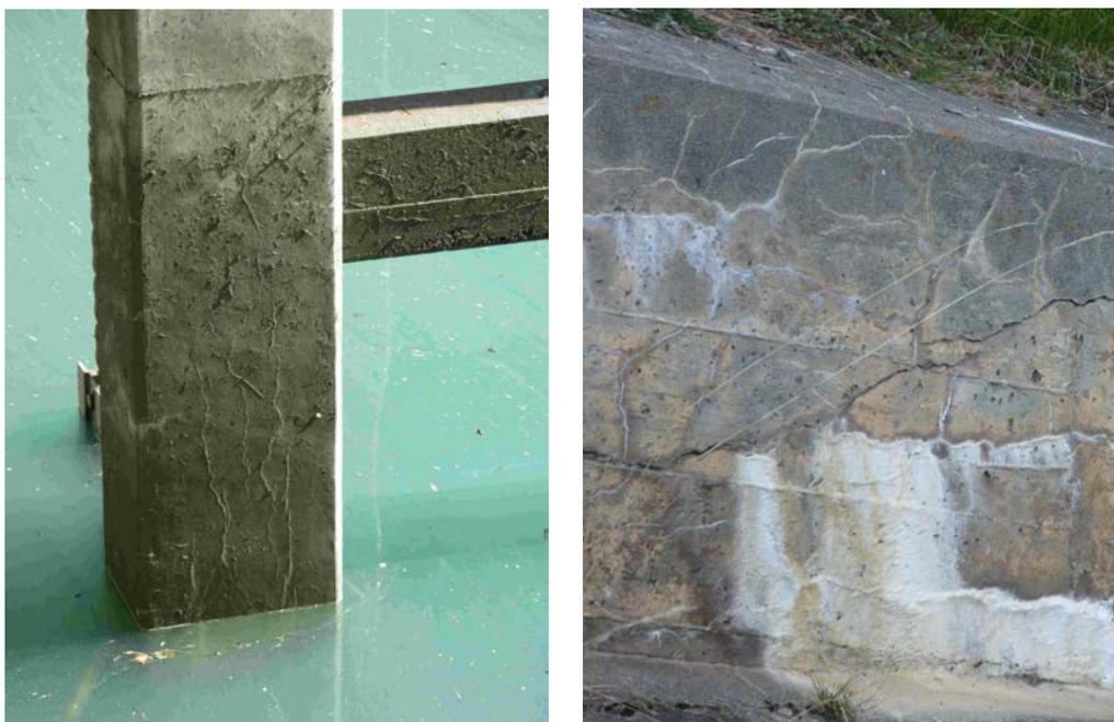
**Figure 16:** Support of a reinforcement bar with AAR cracks in the main vertical stress direction (left) and retaining wall of a surface spillway with gaping crack (right).
