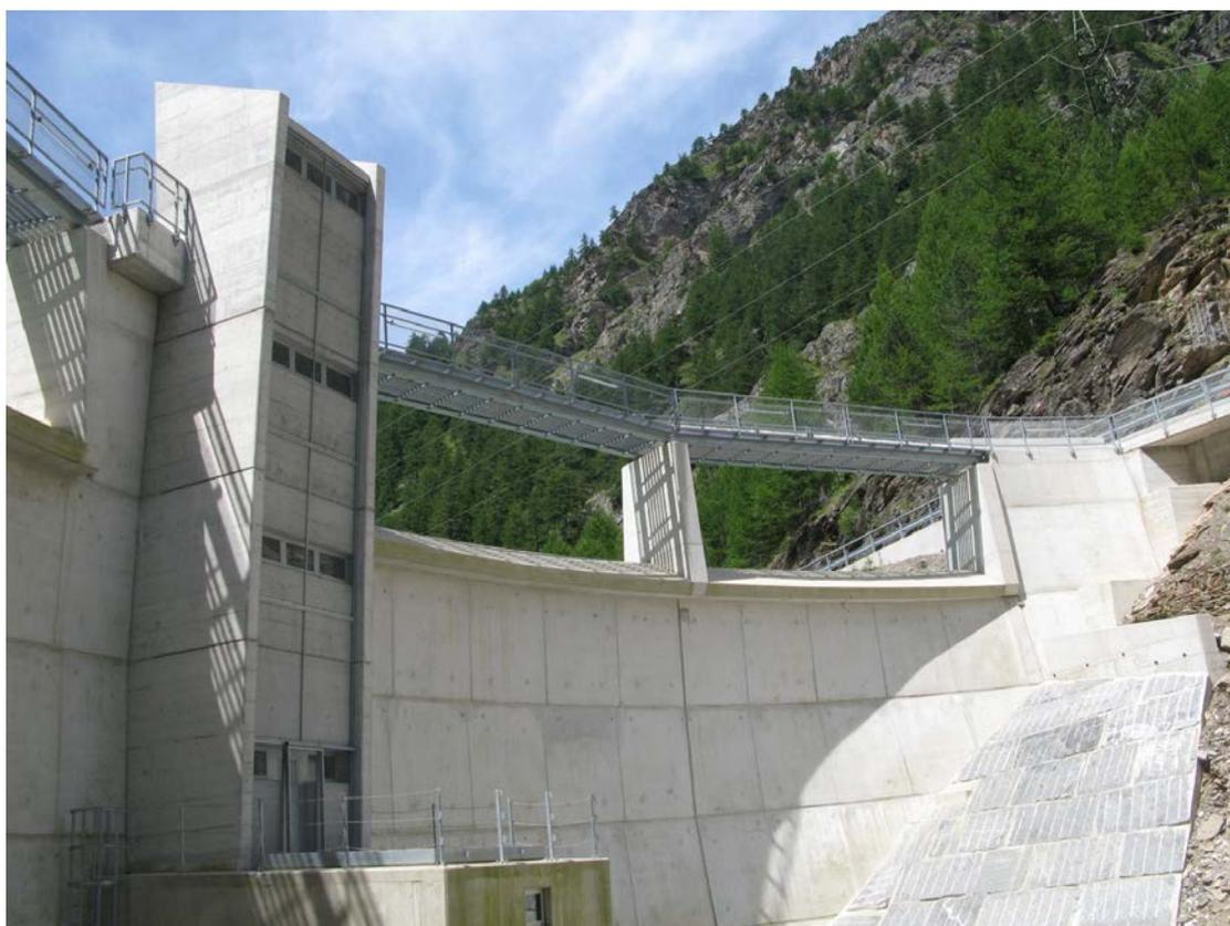
**Figure 22:** Newly constructed Sera Dam in Zwischbergental near Gondo (VS) with non-reactive aggregate concrete [17].
