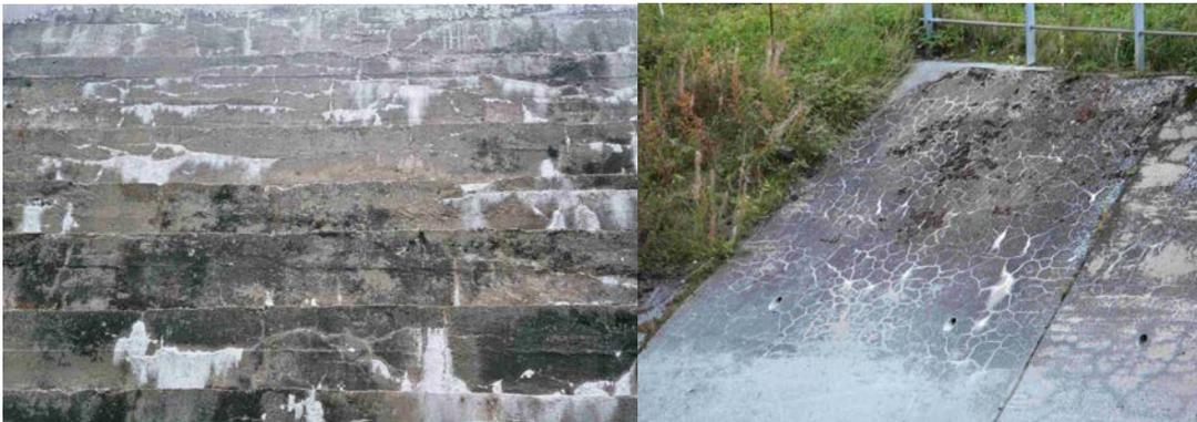
**Figure 13:** AAR cracks with strong air-flow efflorescence at downstream face of a stepped gravity dam (left) and shore protection in the underwater area of a weir with clearly shaped AAR cracks (right).
