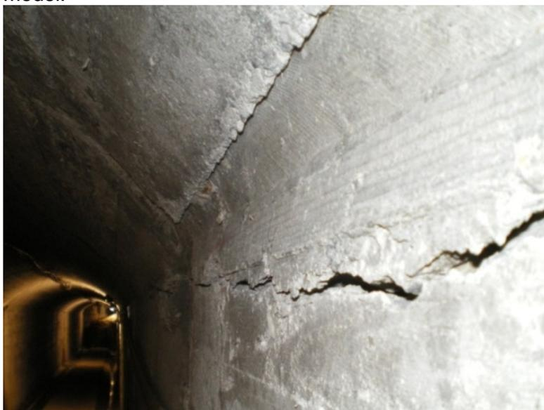
**Figure 77:** Tunnel at the base – Fissuring.
