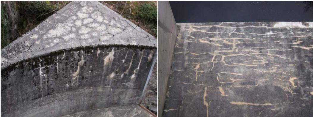
**Figure 12:** Web-shaped AAR cracks at a spillway (left) and cracks at the inlet of a spillway with prevailing crack direction due to existing forces (right).
