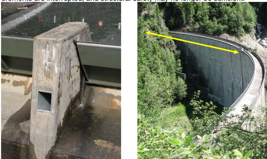
**Figure 17:** Gate mechanisms can no longer be operated due to AAR generated swelling (left) and geodetic monitoring might be interrupted due to AAR rising of the railing on the dam crest (right).
