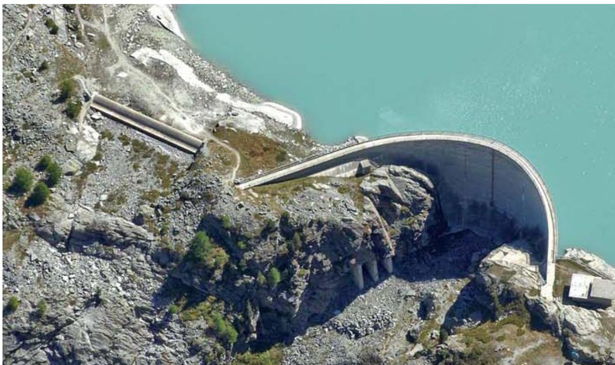
**Figure 58:** Aerial view of Tourtemagne Dam and flood discharge structure on the right bank.
