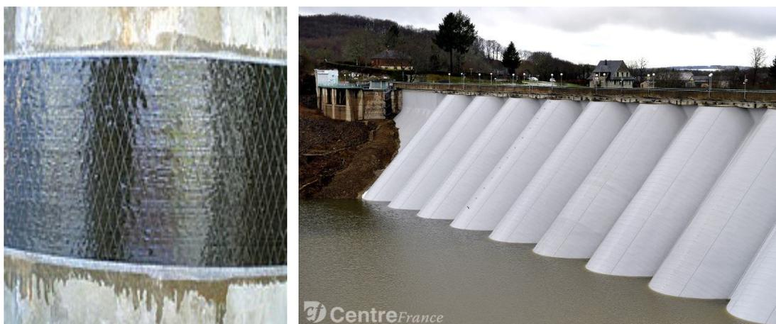
**Figure 83:** Examples of mitigation measures: a) carbon fiber protection; b) protection with PE membrane.
