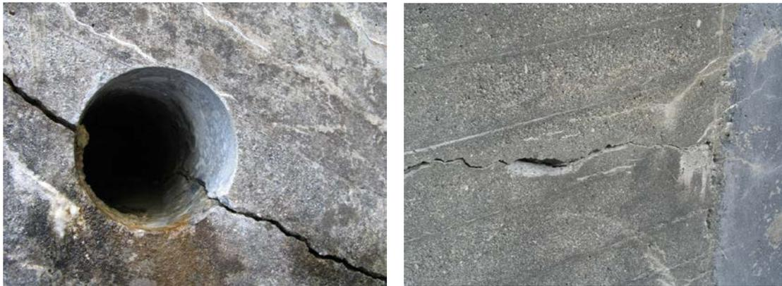
**Figure 18:** Determination of the depth of a structural crack on the downstream face of an AAR affected arch dam by drill core removal (left), and crack with filling on the upstream face of an arch dam.
