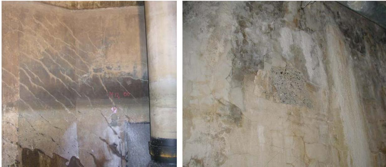
**Figure 61:** Surface condition of certain walls of submerged parts of the power plant.
