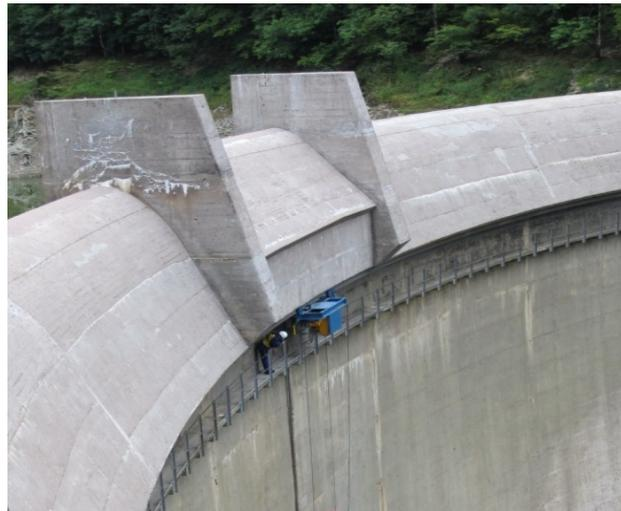
**Figure 54:** View of the guiding walls: horizontal fissuring.
