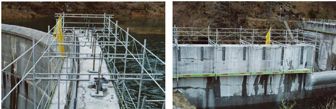
**Figure 19:** Provisional securing of an AAR-damaged dam crest with vertical tensioned anchors, and steel side straps in case of floods and earthquakes.
