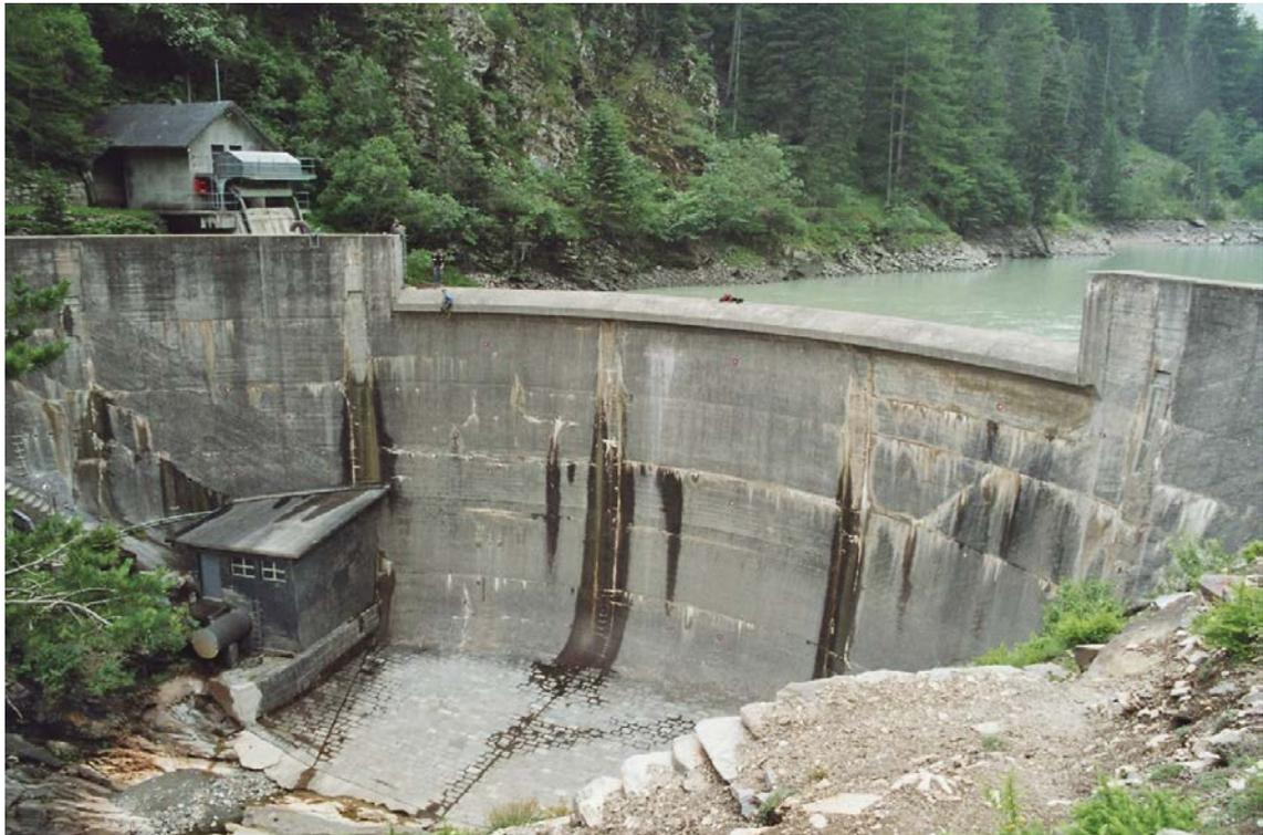
**Figure 1:** Old Sera Dam damaged by AAR at Gondo in Zwischbergental (VS).
